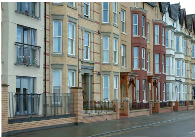
West Parade Existing frontage showing material range
