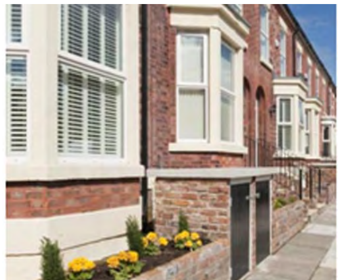
Tancred Street, Liverpool. Example of new frontage design with incorporated bin storage
