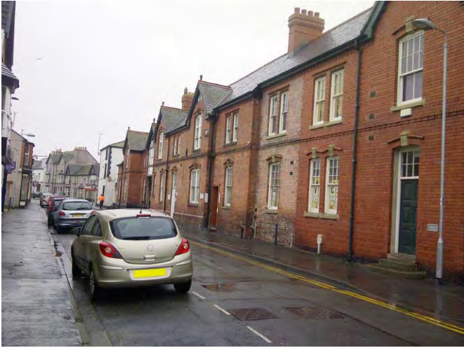
Two storey red brick properties Bedford Street
