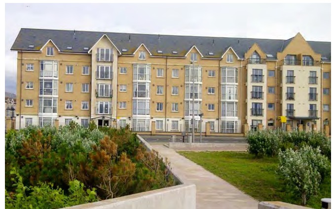
five storey properties West Parade illustrating bay and balcony detailing and contemporary materials
